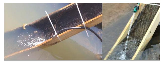
PHOTO 5 EXAMPLES OF ATTRACTION FLOW AT THE BASE OF RAMPS
